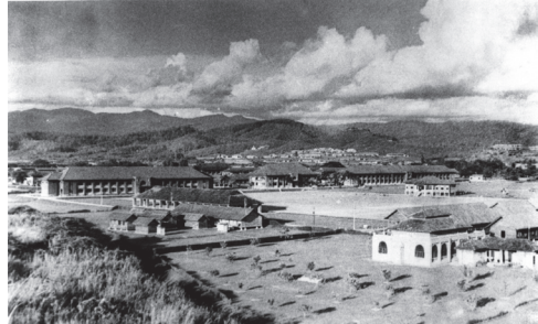
Malayan Police Depot, Jalan Gurney, Kuala Lumpur, (1948–1960) (photo: Department of Information, Kuala Lumpur)
