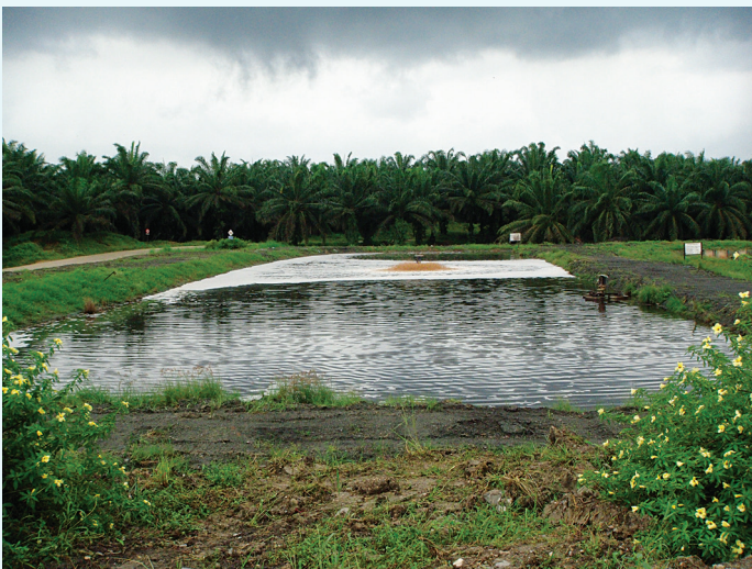
A “Palm Oil Mill Effluent” (POME) lagoon in Sabah. The methane created by these POME lagoons contributes significantly to the palm oil industry’s carbon footprint. Photo credit: Oliver Pye, 2011.
