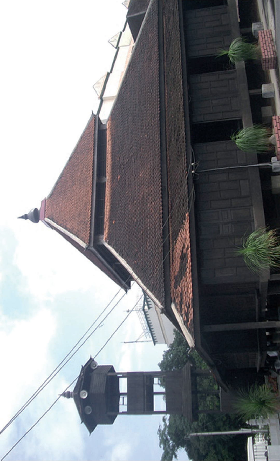
M11. The oldest mosque in Kelantan, Masjid Kampung Laut at Nilam Puri, Kota Bharu, Kelantan, was built with a multi-tiered roof in the 1730s. Photo taken by the author.
